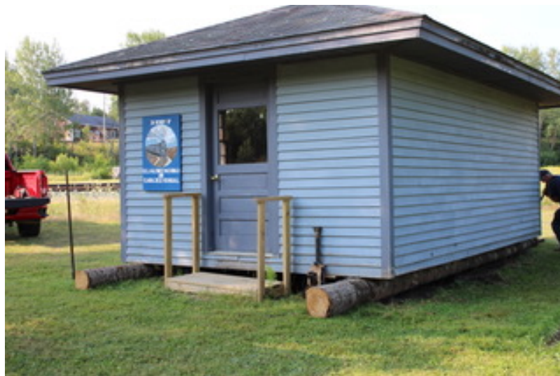
Preparing the railroad museum for the move
